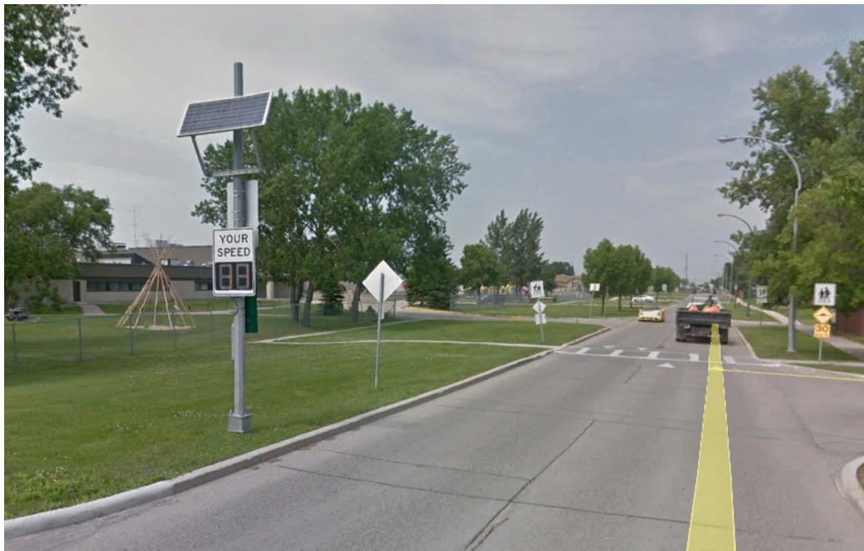
Figure 2: Speed Reader Board and Raised Crosswalk Installation at Bernie Wolf School on Bournais Drive (Photo Source: Google Street View)
